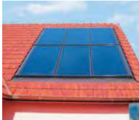
Abb. B.1.6–8 Indachmontage
